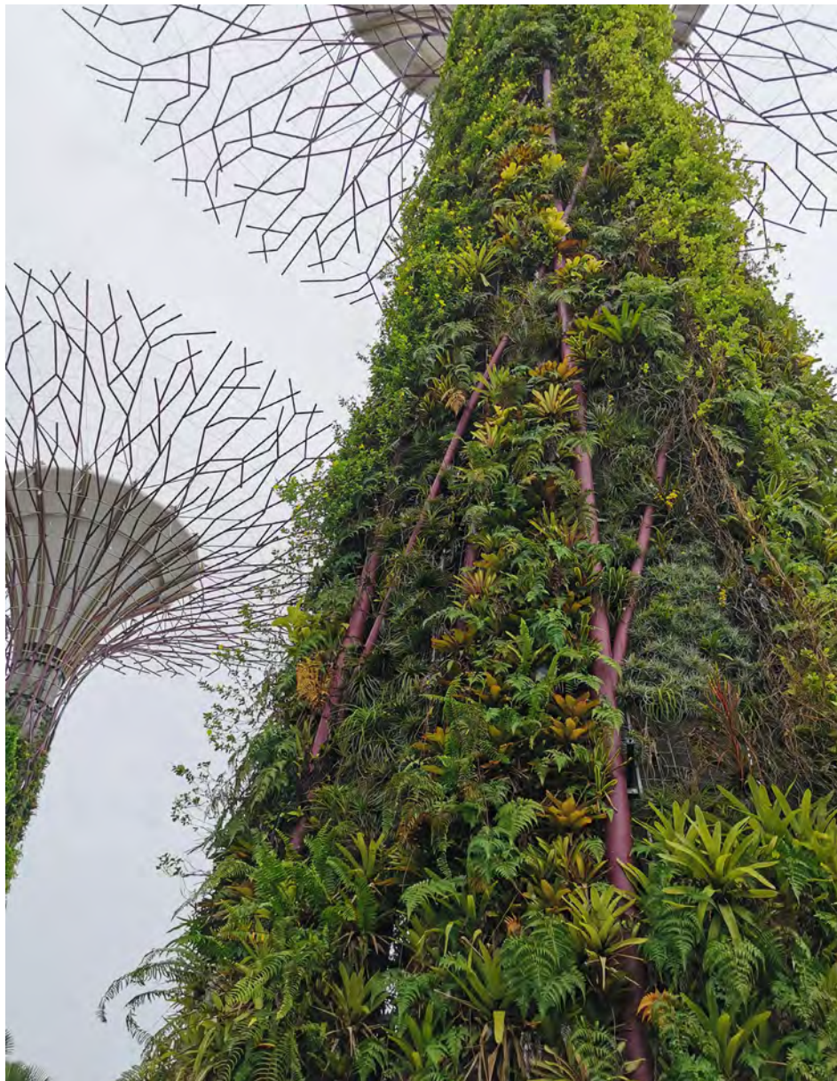
Figure 2: View upwards of one of the Super Trees. The solar photovoltaic cells are integrated into the inverted canopy structure at the top of the tree. 11 out of 18 trees have these photovoltaic systems.
