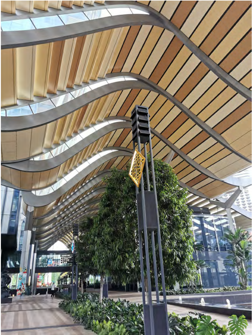
Figure 3: View from the first seated observation area. In the foreground of the image is an orange-coloured, covered walkway with integrated solar cells (known as solar ‘canopy-ribbons’) joining residences, a hotel, and an office complex. In the background, the walkway continues to join a service node: the underground metro service, a commercial services area (F&B establishments), a play area, and a rest area.
